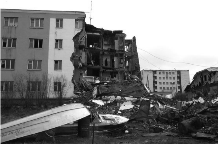
Figure 12.7. Collapsed apartment building in Cherskii, northern Siberia. Sections of the building collapsed as underlying permafrost melted. (Image courtesy of Professor V. E. Romanovsky, University of Alaska, Fairbanks)
