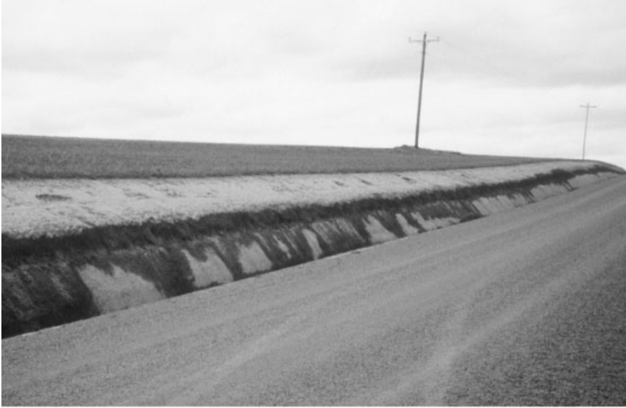
Figure 8.7. Effect of a fragipan on near-surface hydrology in a cultivated Fragixeralf landscape in northern Idaho. A seasonal perched water table above the fragipan appears as the dark layer in the road cut. Much of the incident precipitation is shed from these hillslopes as lateral throughflow.
