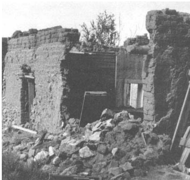
Fig. 8.3. The collapse of an adobe wall created a large sedimentary deposit outside this structure at Concho, Arizona.
