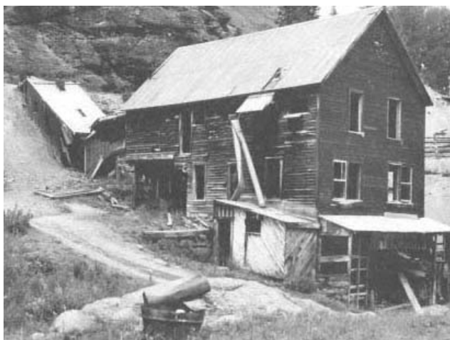
Fig. 5.3. Abandoned structure, largely unscavenged, in the "ghost town" of Sneffels, Colorado.
