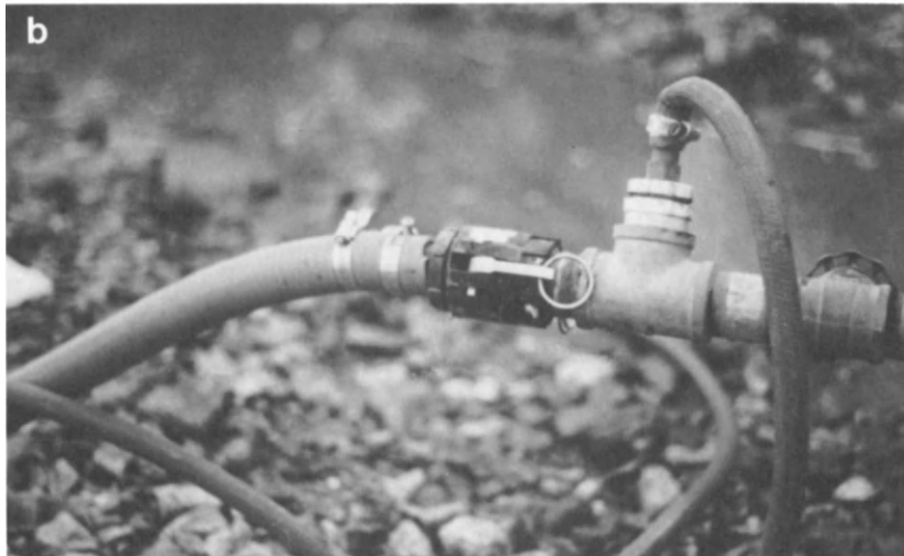
Figure 2.23 In a SMAP-style flotation system, (a) water is pumped from a water source, such as a stream, directly into the barrel; a gasoline-powered pump is commonly used. A shut-off valve (b) regulates water flow and allows water to be diverted to a small-diameter hose used for washing equipment.
