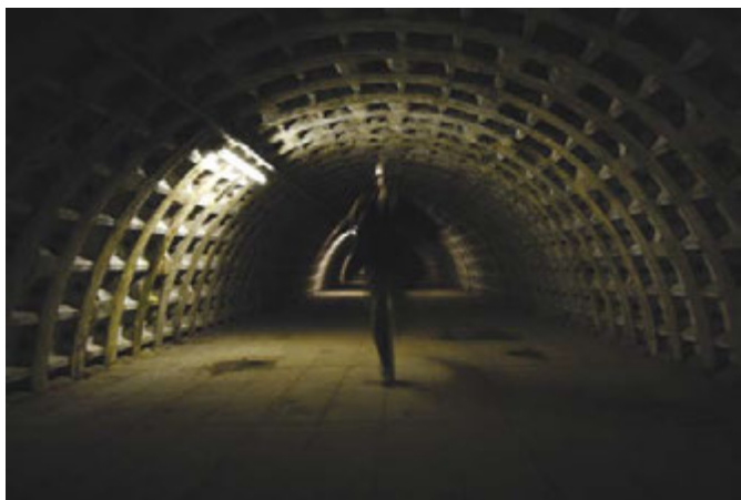
FIGURE 14.1 Speciation in mosquitoes in the London Underground. A large, deep shelter built alongside London's Underground subway system. This is an ideal breeding ground for the mosquito Culex pipiens molestus .
