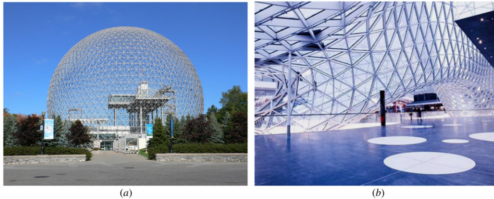
Figure 2. (a) Geodesic Dome Montreal 1967, Buckminster Fuller (photo: Philip Hienstorfer). (b) Grid Shell Frankfurt MyZeil, Architect: M Fuksas, Rome; Engineer: Knippers Helbig Advanced Engineering (Knippers and Helbig 2007, 2009; photo: Christian Sauter).
