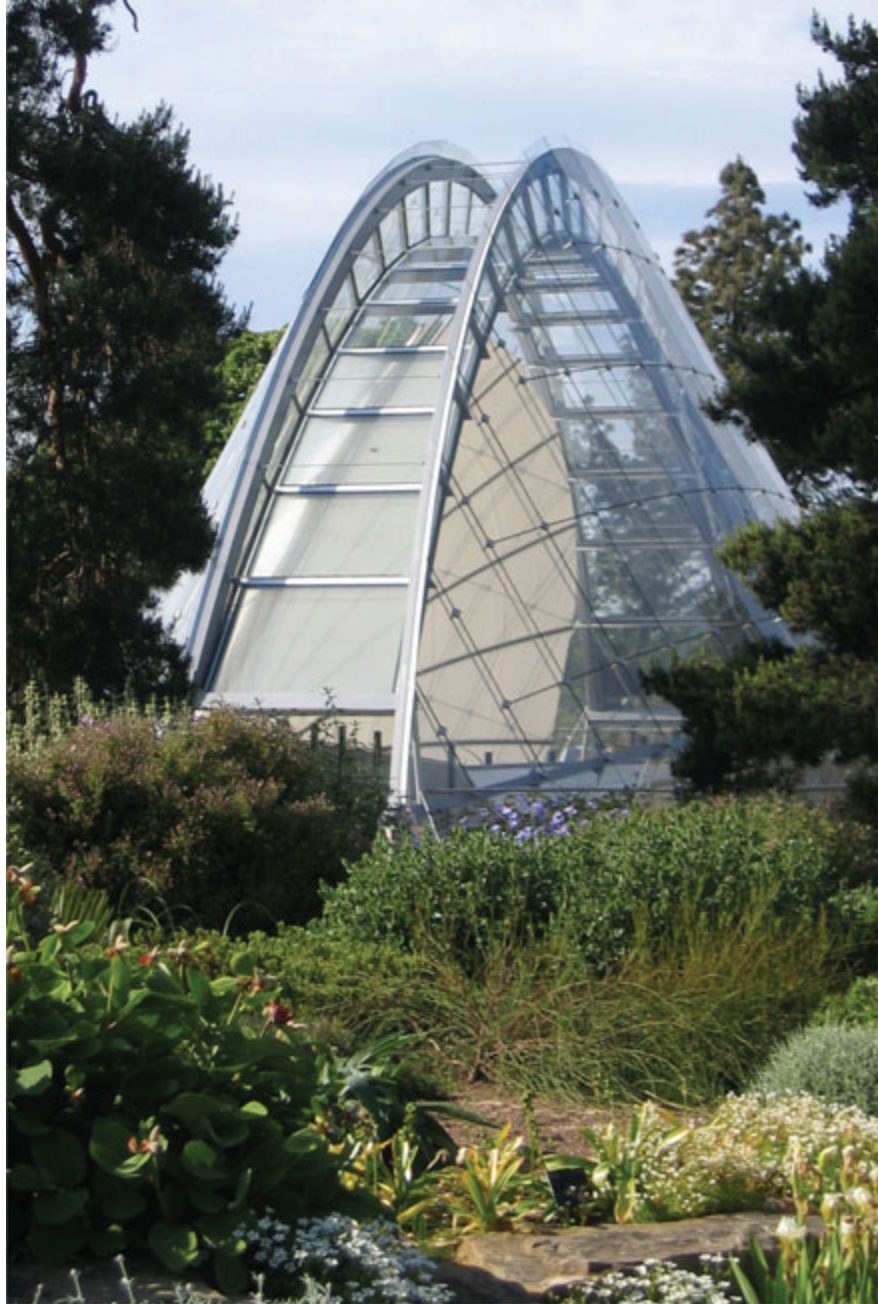
120 . The Davis Alpine House at Kew Gardens by Wilkinson Eyre and Atelier Ten. Ideas from termite mounds were employed to create the cool conditions necessary for the collection of alpine plants
