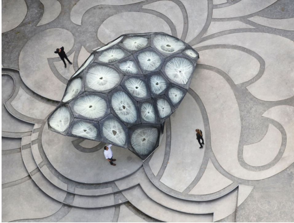
91 . The ICD/ITKE Research Pavilion at the University of Stuttgart, made from robotically woven fibres based on a detailed understanding of the morphology of beetle shells
