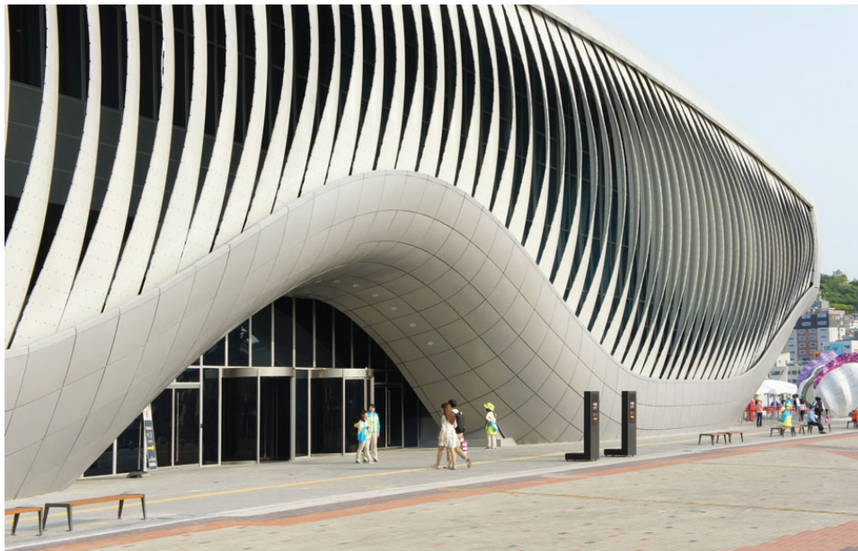
115 . Thematic Pavilion by soma, using a kinematic facade inspired by early research on the flectofin as a dynamic part of the facade that controls solar gain
