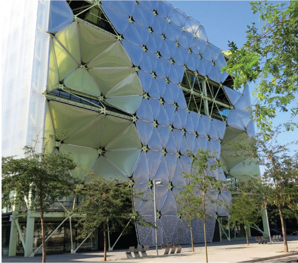
124 . Media-TIC by Cloud 9 – using a wide array of sensors and adaptive facades together with renewable energy generation to deliver a near net zero energy building
