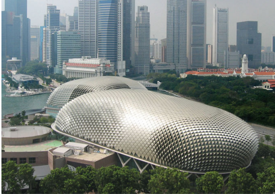
113 . The Singapore Arts Centre, designed by Atelier One, Atelier Ten and Michael Wilford & Partners, showing what can be achieved with shading systems based on plants
