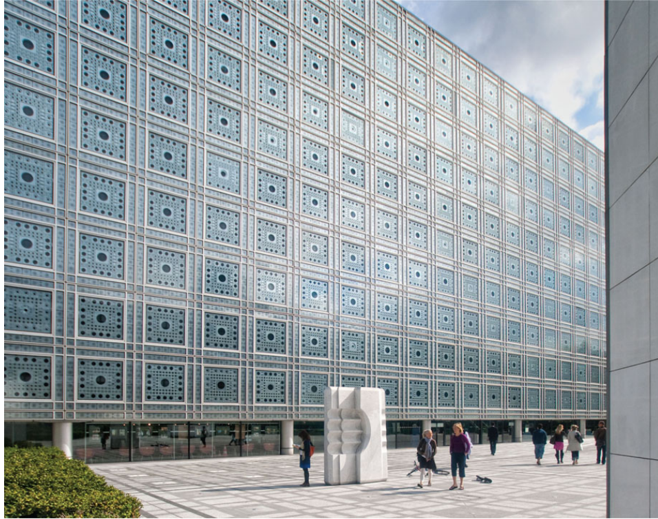
122 . The facade of the Institut du Monde Arabe by Jean Nouvel – a climate-adaptive building skin that also has cultural references to the mashrabiya of vernacular Middle Eastern architecture
