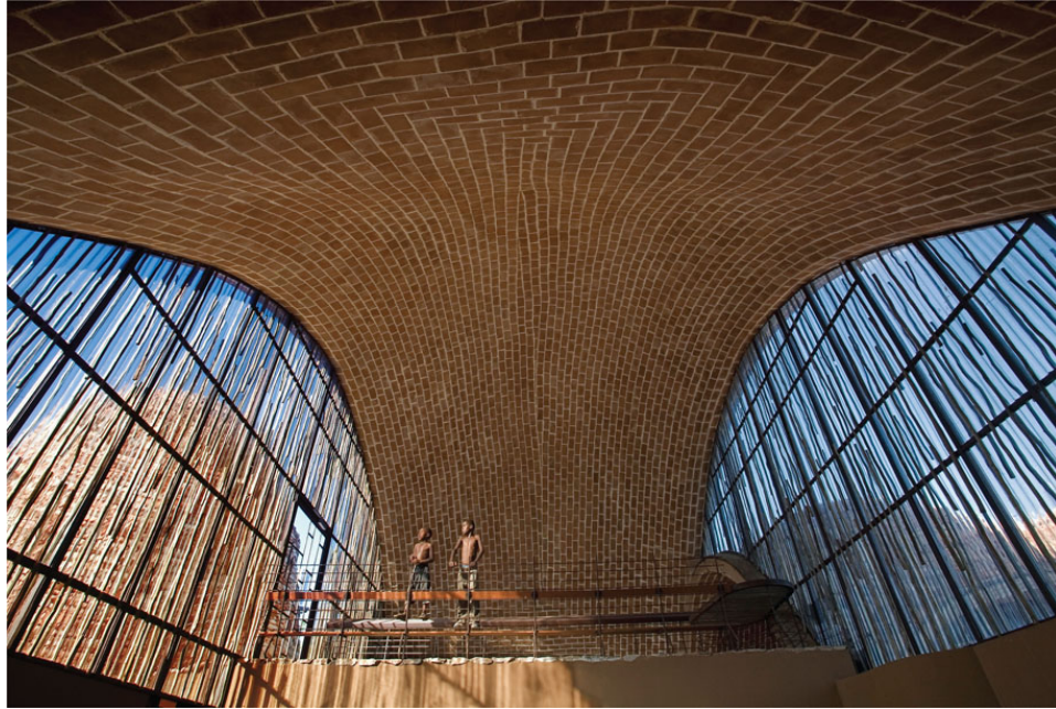
23 . Mapungubwe Interpretation Centre designed by Peter Rich Architects using Guastavino vaulting – similar to an abalone shell and made with basic materials, such as sun-baked earth tiles
