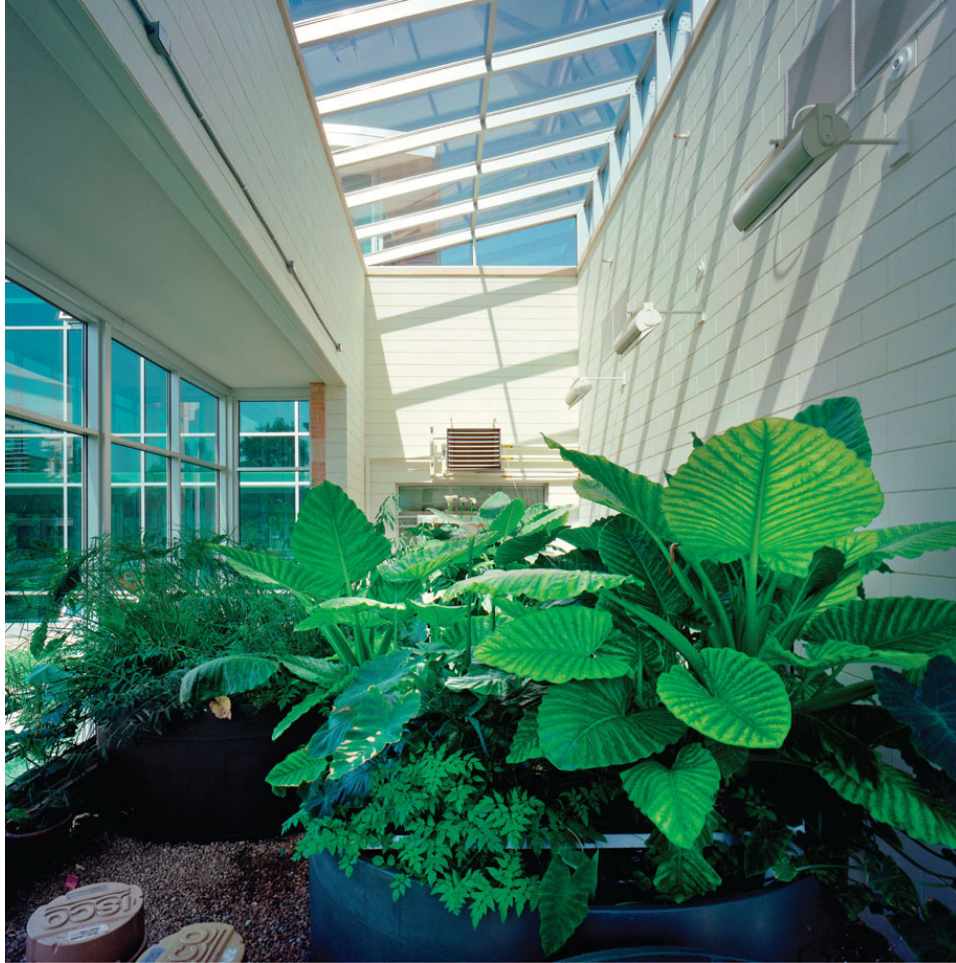
110 . A Living Machine®, at the Adam Joseph Lewis Center for Environmental Studies, Oberlin College by William McDonough + Partners, that uses plants and micro-organisms to treat waste water
