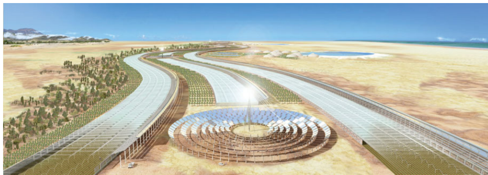
138 . Sahara Forest Project (SFP) – a scheme that integrates horticulture, forms of solar energy and desert revegetation to deliver numerous synergies and secondary benefits
