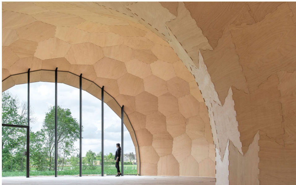
36 . Landesgartenschau Exhibition Hall at the University of Stuttgart – made from interlocking plywood panels based on the structure of a sea urchin skeleton
