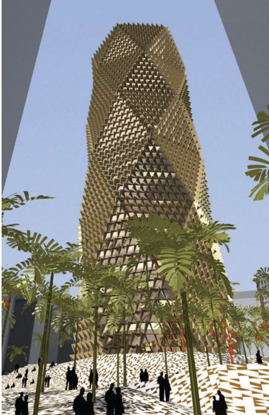
112 . Cabo Llanos Tower masterplan in Santa Cruz de Tenerife, Spain, by Foreign Office Architects – with palm-leaf inspired shading fins that follow the movement of the sun
