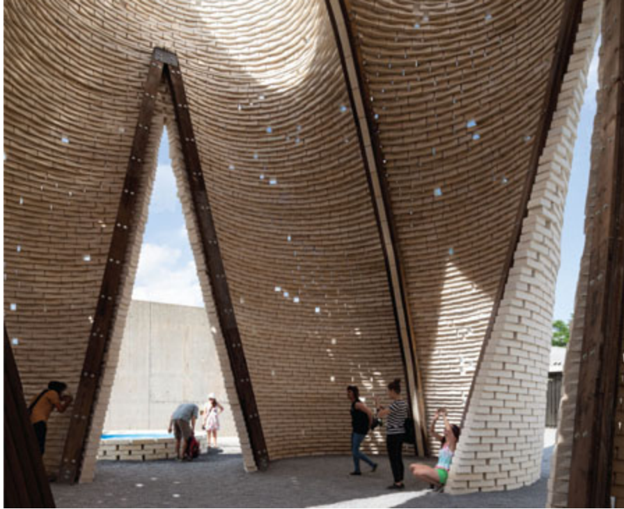
78–79 . ‘Hy-Fi’ by The Living, constructed using bricks that were grown using fungal mycelia
