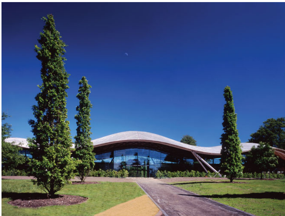
24 . The Savill Building by Glenn Howells Architects. By using small sections of timber in a highly efficient form, gridshells can achieve factor-15 savings in resource use
