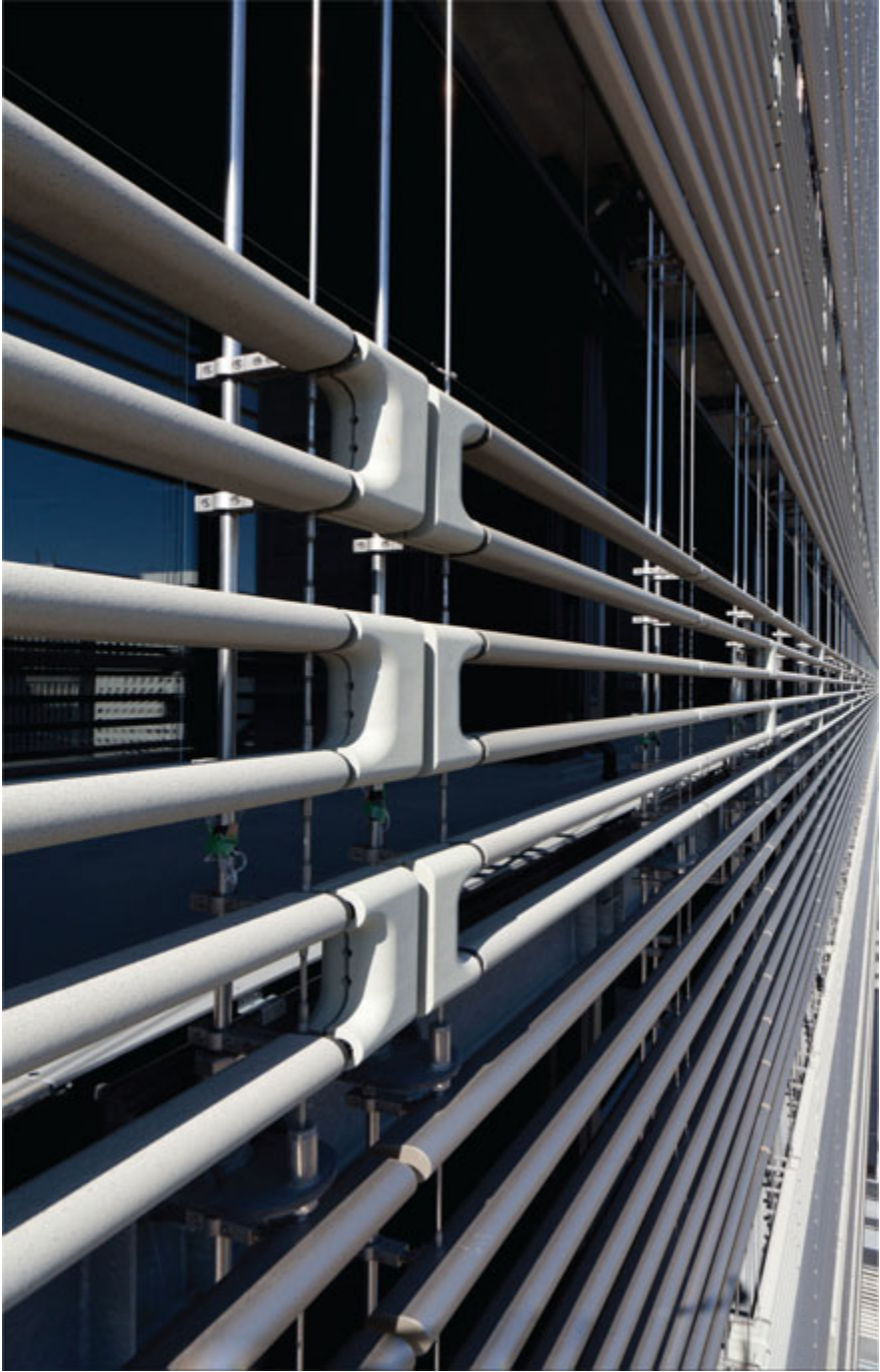
123 . Nikken Sekkei's BioSkin, which delivers evaporative cooling from harvested rainwater to modify its microclimate
