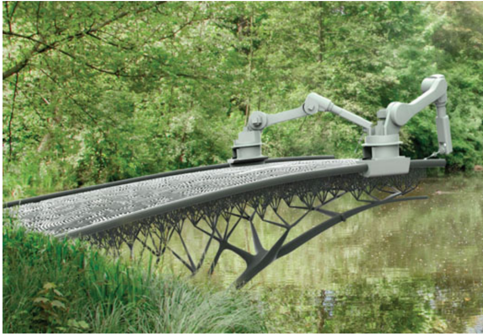
12. 3D-printed bridge by Joris Larman Lab demonstrating the expressive and material-efficient results of designing with SKO software
