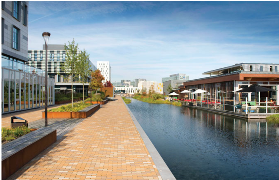
99 . The Biological Nutrient Pavilion at Park 20/20, providing fresh food (partly grown on site) as part of the biological cycle for the site, as well as benefitting from the visual amenity of a creatively designed water cycle
