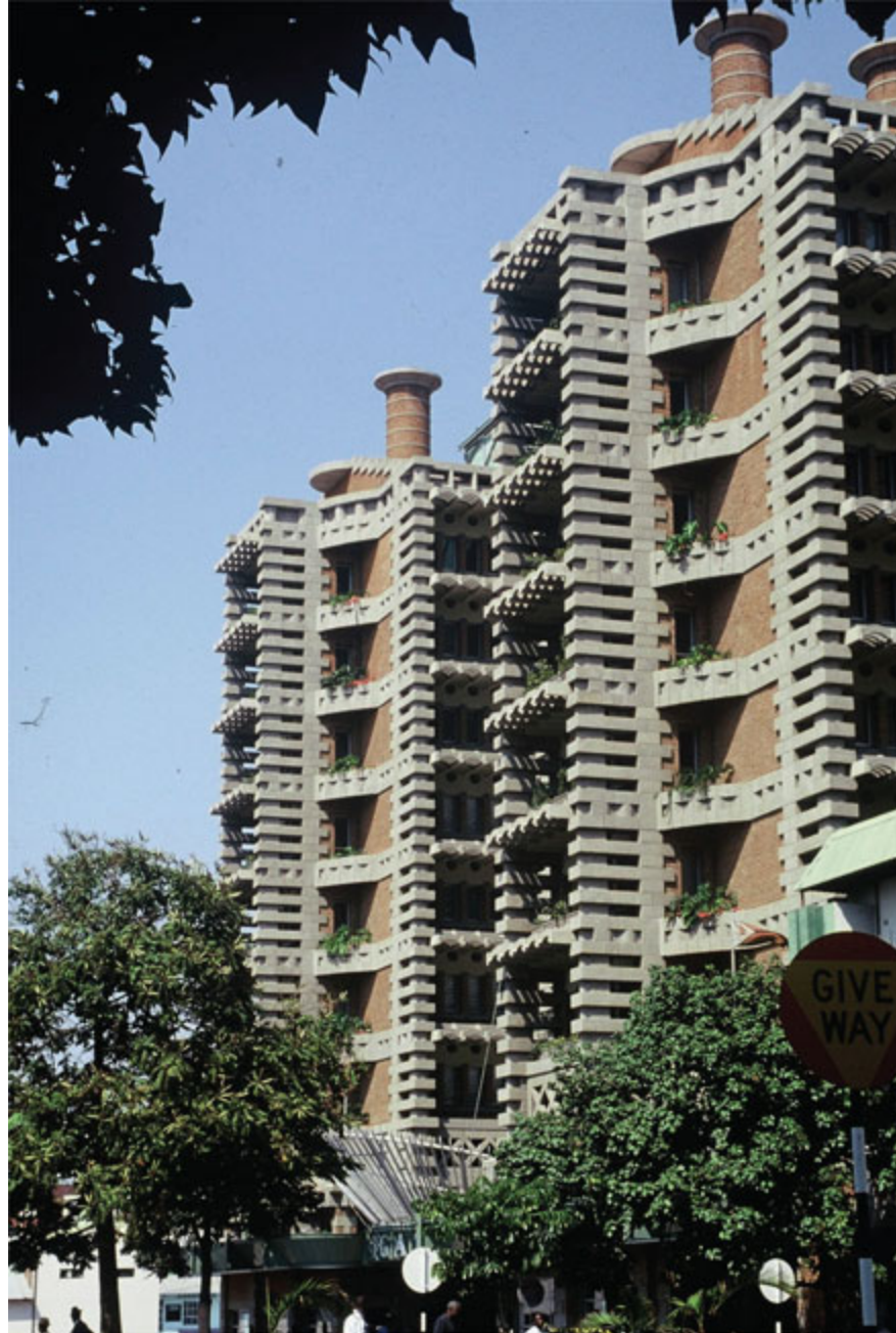
119 . The Eastgate Centre by architect Mick Pearce – a building inspired by termite mounds that maintains comfortable conditions close to the equator without mechanical cooling
