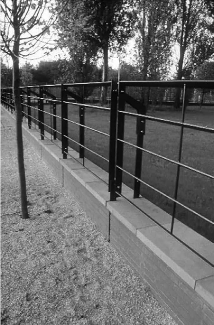
Figure 3.2 Fencing in Hulme Park, Manchester (UK).
