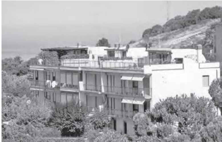
Figure 9.19 View of the building. Courtesy of Elsevier.
