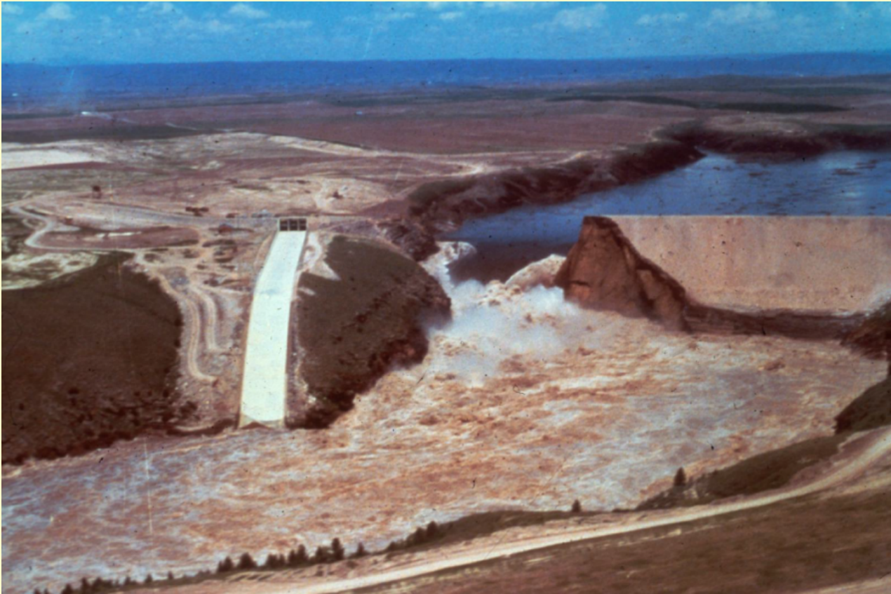
Teton Dam failure
