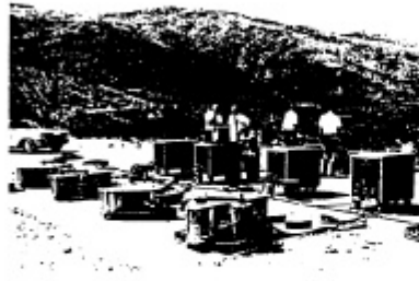
Fig. 7.9. Four synchronous vibration generators exciting an earth-filled dam. (From Kojima, 1966.)
