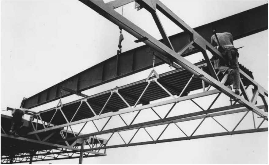
Figure 1.17 Steel deck is designed as top chord of prefabricated open web steel joists. ( Inland-Ryerson Construction Products Company. )
