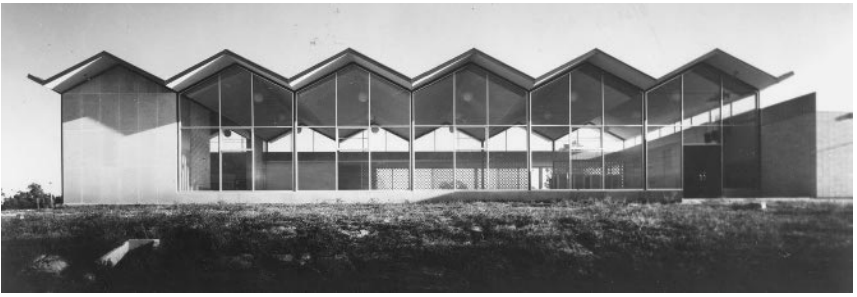
Figure 9.14 Cold-formed steel panels used in folded-plate roof. ( H. H. Robertson Company. )
