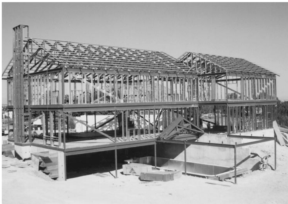
Figure 14.1 Cold-formed steel framing used for housing. ( Elliott Steel Homes, Inc., Loveland, CO )
