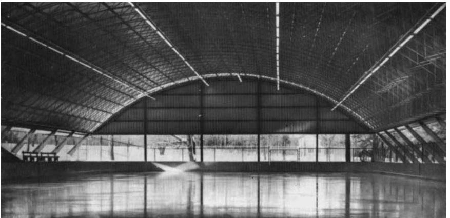
Figure 1.8 Cold-formed steel members used in a 100 \times 220 \times 30 -ft ( 30.5 \times 67.1 \times 9.2 -m) triodetic arch. ( Butler Manufacturing Company. )
