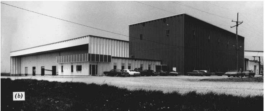
Figure 1.18 (a) Exterior curtain wall panels employing corrugated steel sheets. 1.87 (b) Frameless stressed-skin construction ( Behlen Manufacturing Company. )
