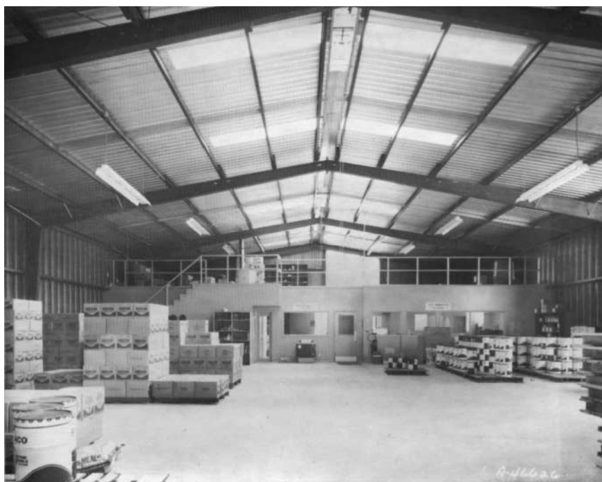
Figure 1.21 Standardized building made of fabricated rigid frame with cold-formed sections for girts, purlins, roofs, and walls. ( Armco Steel Corporation. )
