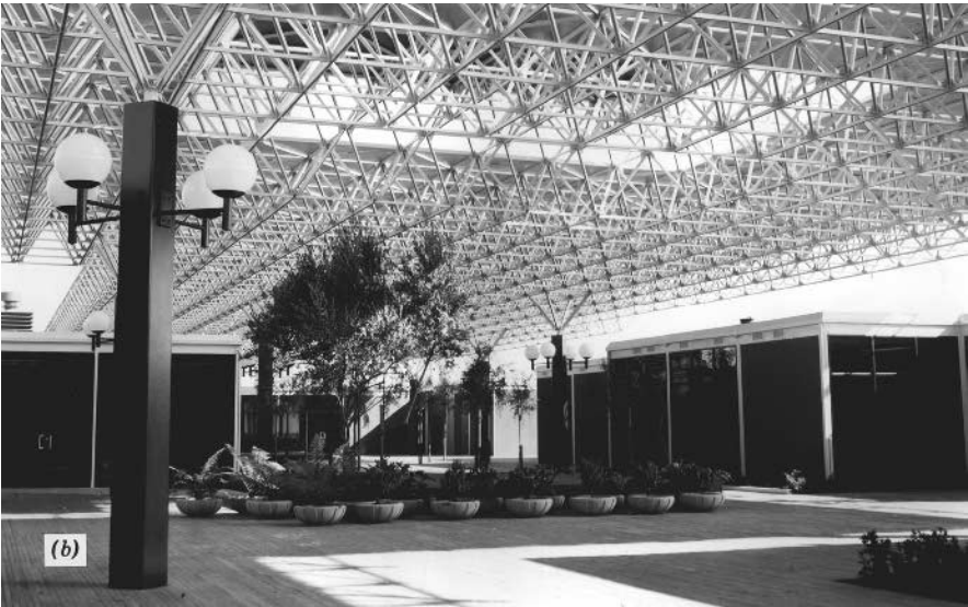
Figure 1.6 Cold-formed steel sections used in space frames ( Unistrut Corporation. )
