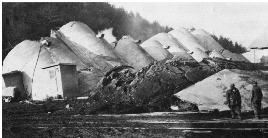
Fig. 3.3 Bearing capacity failure of a silo foundation. (From Tschebotarioff, 1951.)
