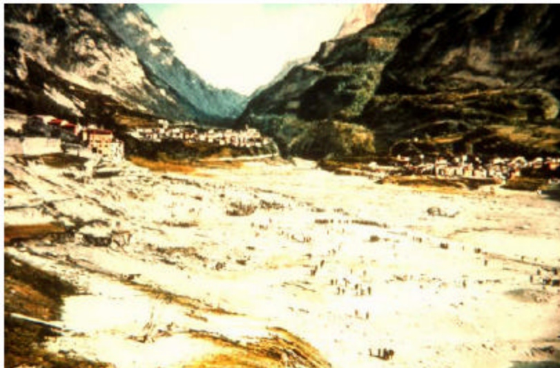
Figure 1.1d: The remains of the town of Longarone after the flood caused by the overtopping of the Vajont dam as a result of the Mount Toc failure. More than 2000 persons were killed in this flood.
