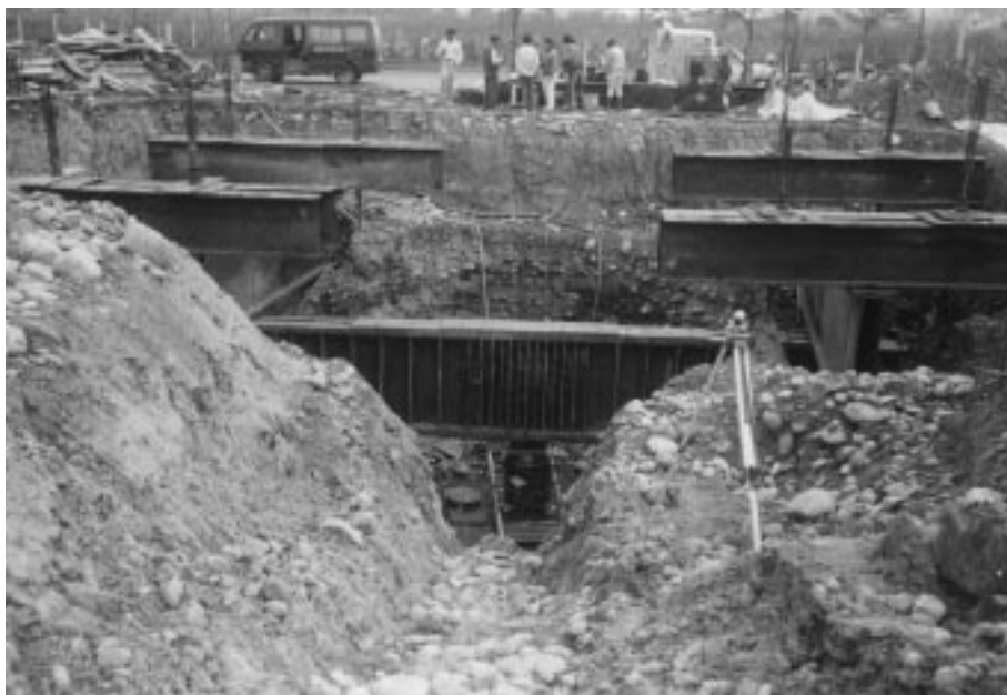
Fig. 7. Complete setup for the plate-load test.
