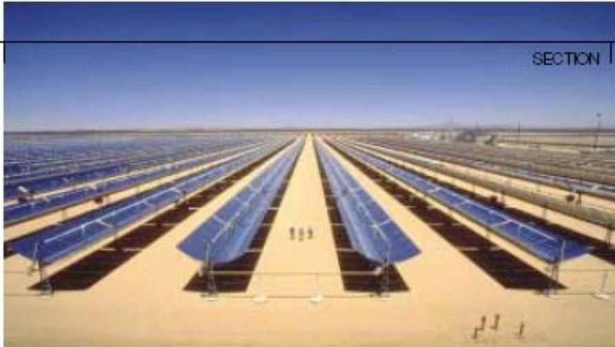
Figure 4 Parabolic trough concentrating solar collector field of the 150 MW (5 x 30 MW) steam cycle solar electricity generating systems at Kramer Junction, California (Source: KJC)
