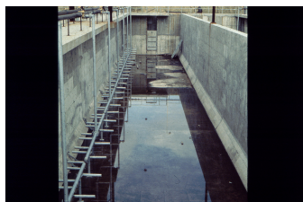
Empty basin showing aeration manifold
