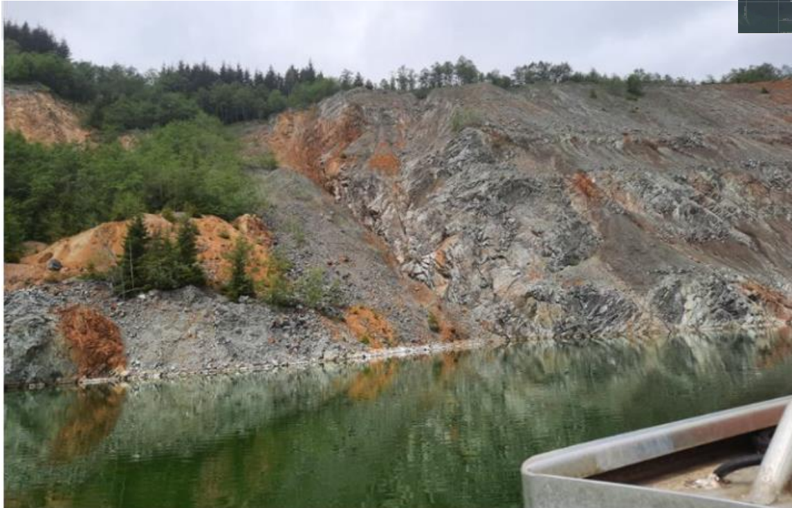
West slope movement (north end)
