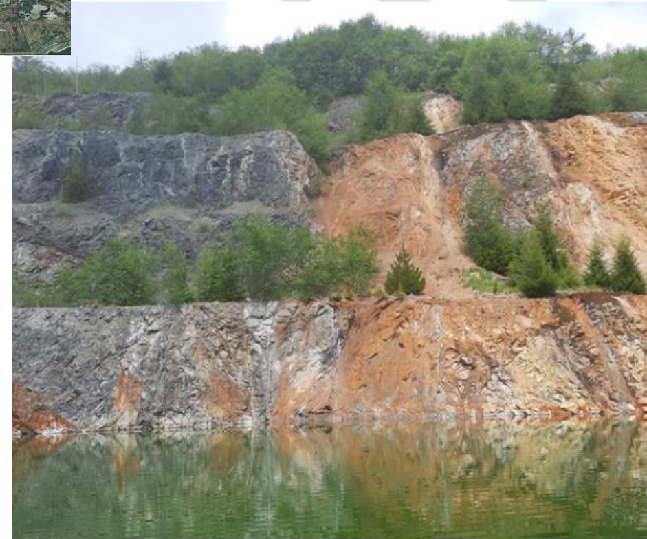
North wall slide
