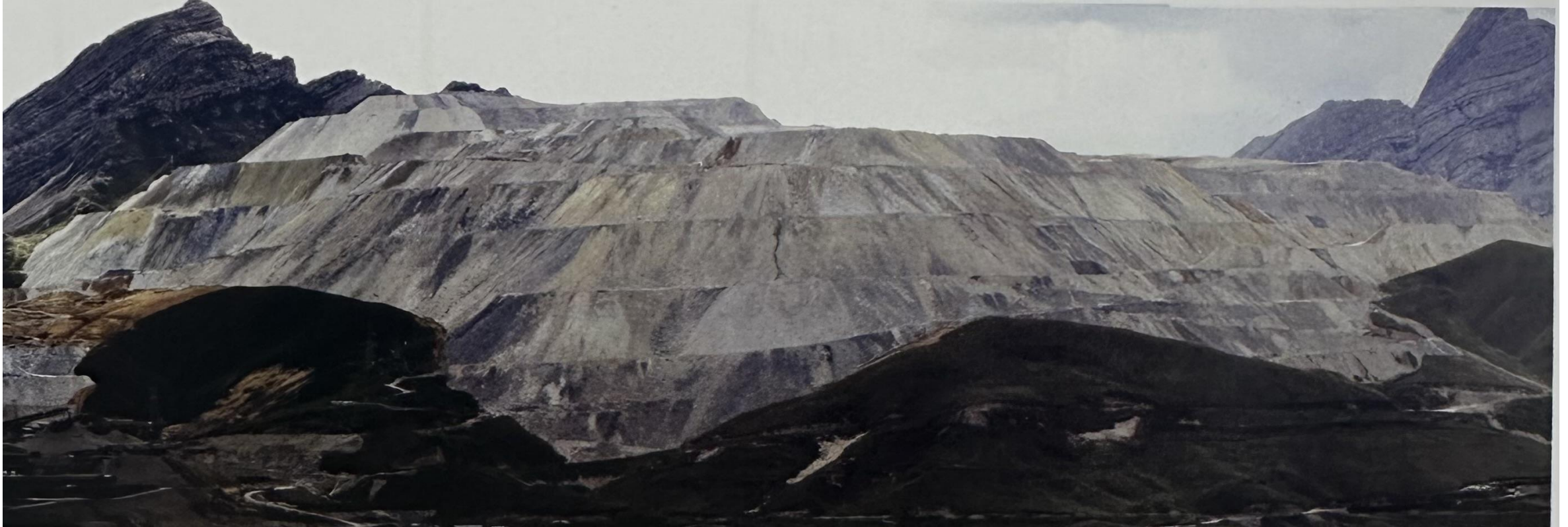
East Dump at the Antamina Mine, Peru, 2010 (Guidelines for Waster dump and Stockpile design, 2017)
