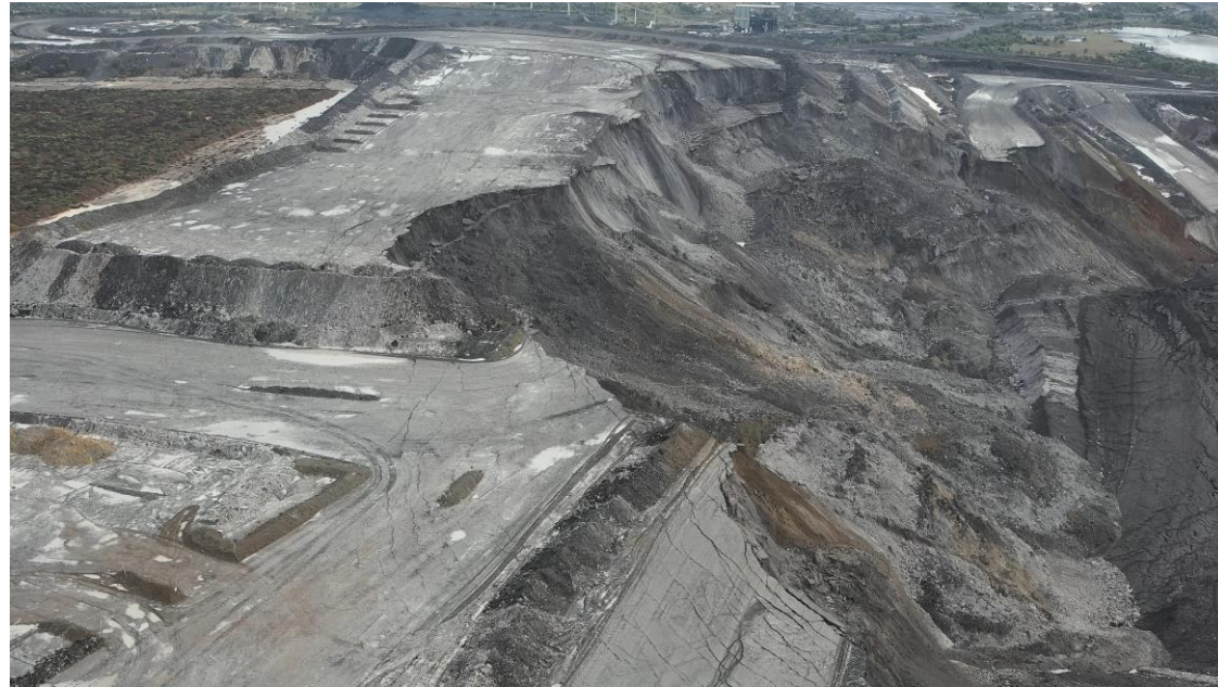
Spoil dump failure
