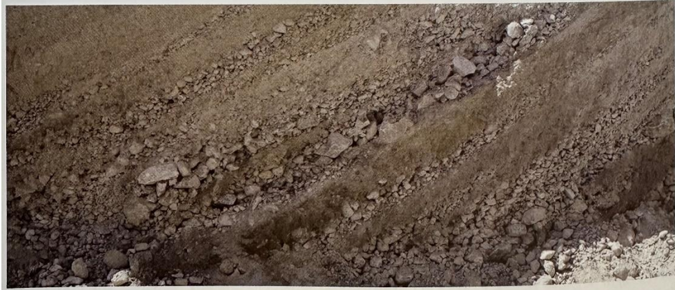
Illustration of piping along internal preferential flow pathways
