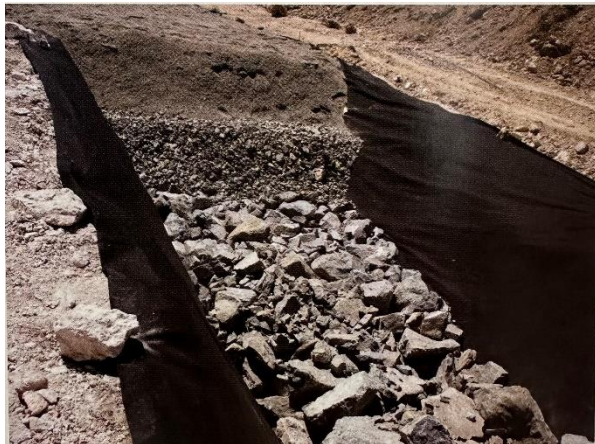
Rock drain under construction showing drain rock and granular filters
